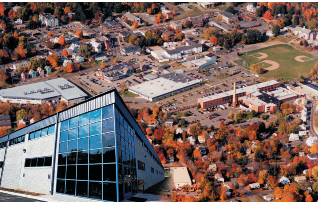
Siemon's Watertown, CT-based Global Headquarters and North American Manufacturing Facility.
